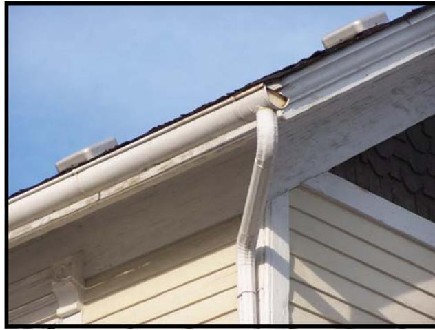
*Half-round gutters with rounded downspouts*
