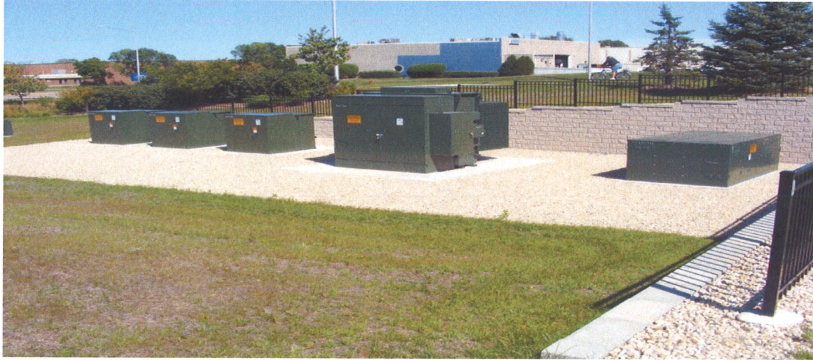
LDC-1 with the 35 kV gear, the 35 kV to 12 kV dead front transformer and the single phase regulators from right to left above.
