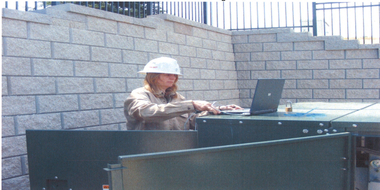
St Charles Substation Engineer, Erika Drennen, uses a laptop to program the relays in the control enclosure attached to the 35 kV gear.
