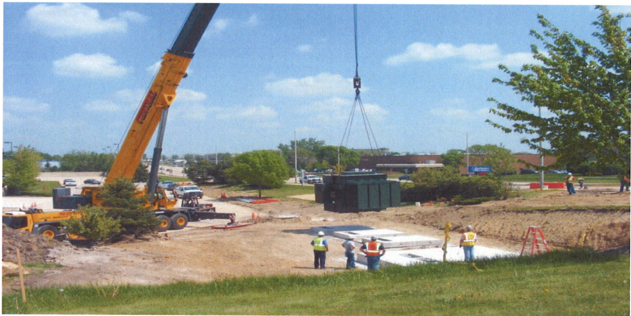
The crew watches as the 34.5 kV to 12.47 kV 10 MVA dead front transformer approaches the precast concrete pad.
