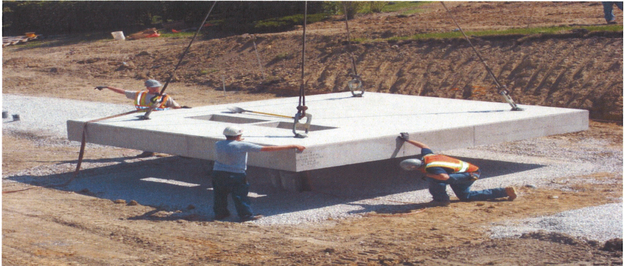
The 50,000 lb transformer pad was set just minutes before the transformer.
