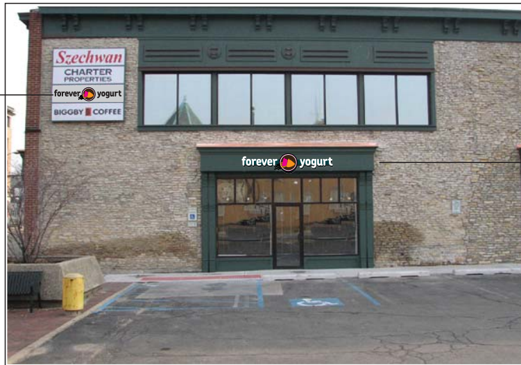
WEST ELEVATION AT 117 W. MAIN ST.
