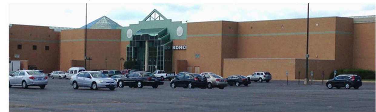
Existing Mall Facade "Draft not for Public Dissemination"
