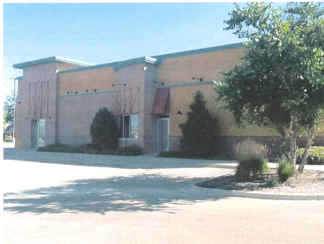
EXISTING SIDE ENTRANCE
