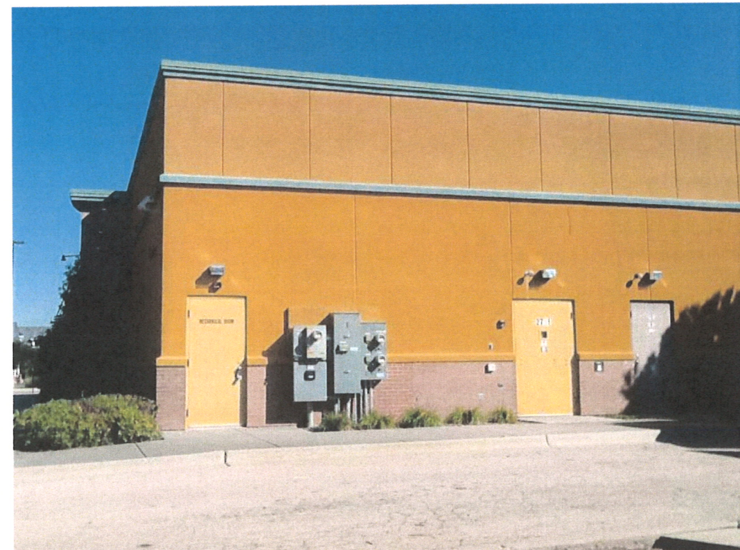
EXISTING REAR EXIT
