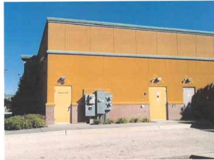
EXISTING REAR EXIT
