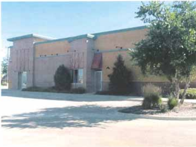
EXISTING SIDE ENTRANCE
