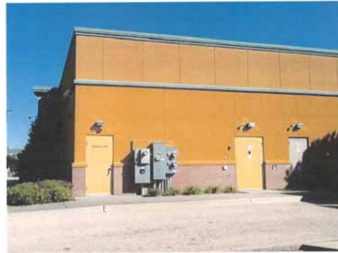
EXISTING REAR EXIT
