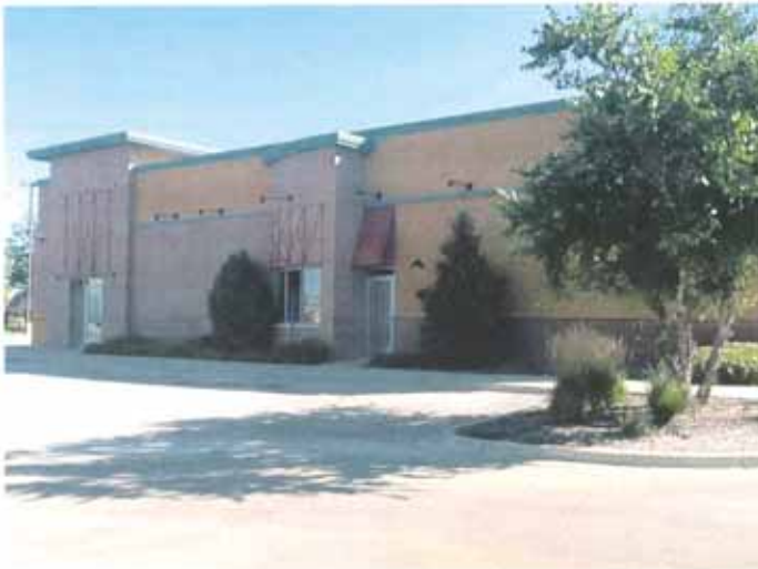
EXISTING SIDE ENTRANCE
