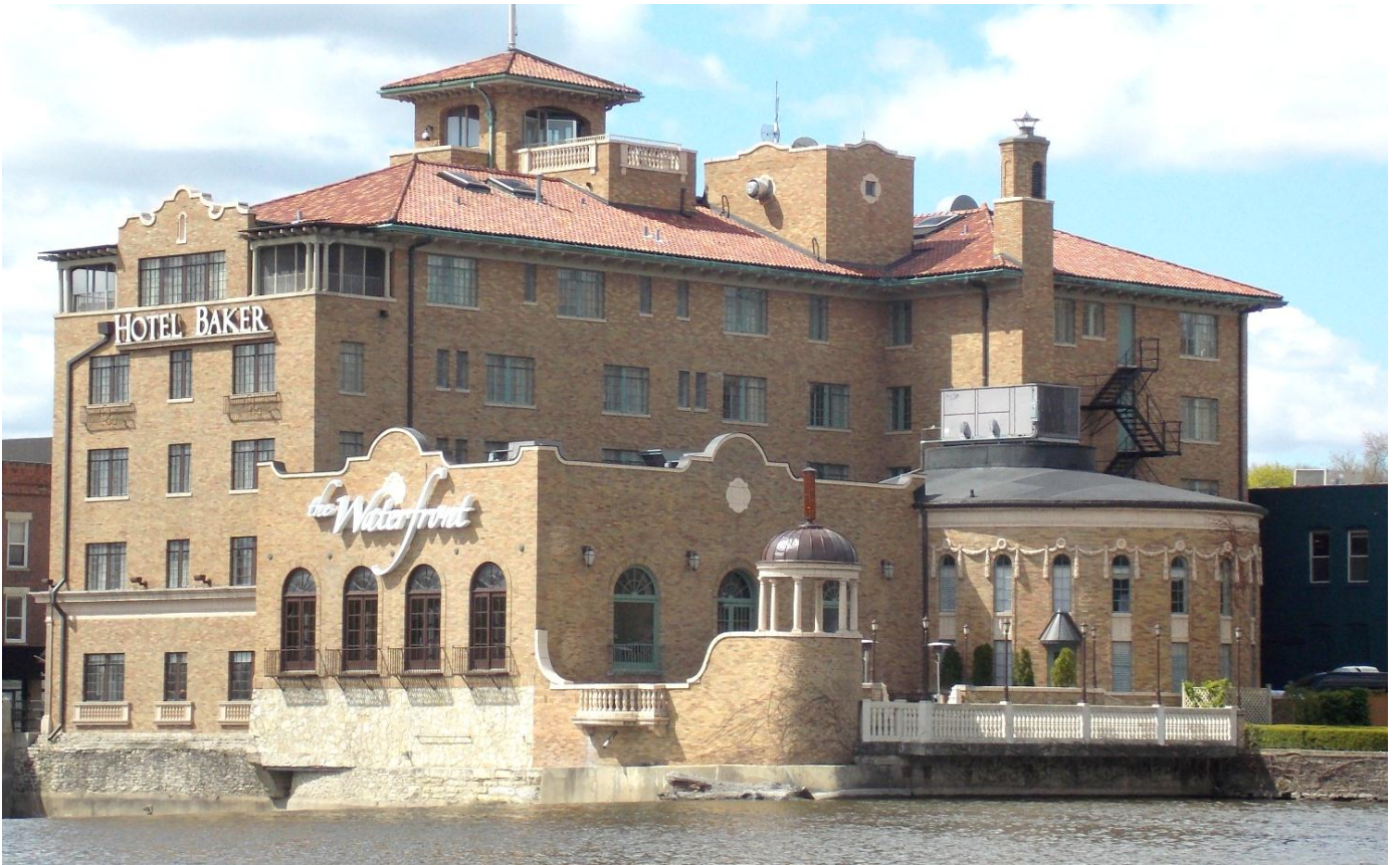
Hotel Baker – North Elevation (rear)
