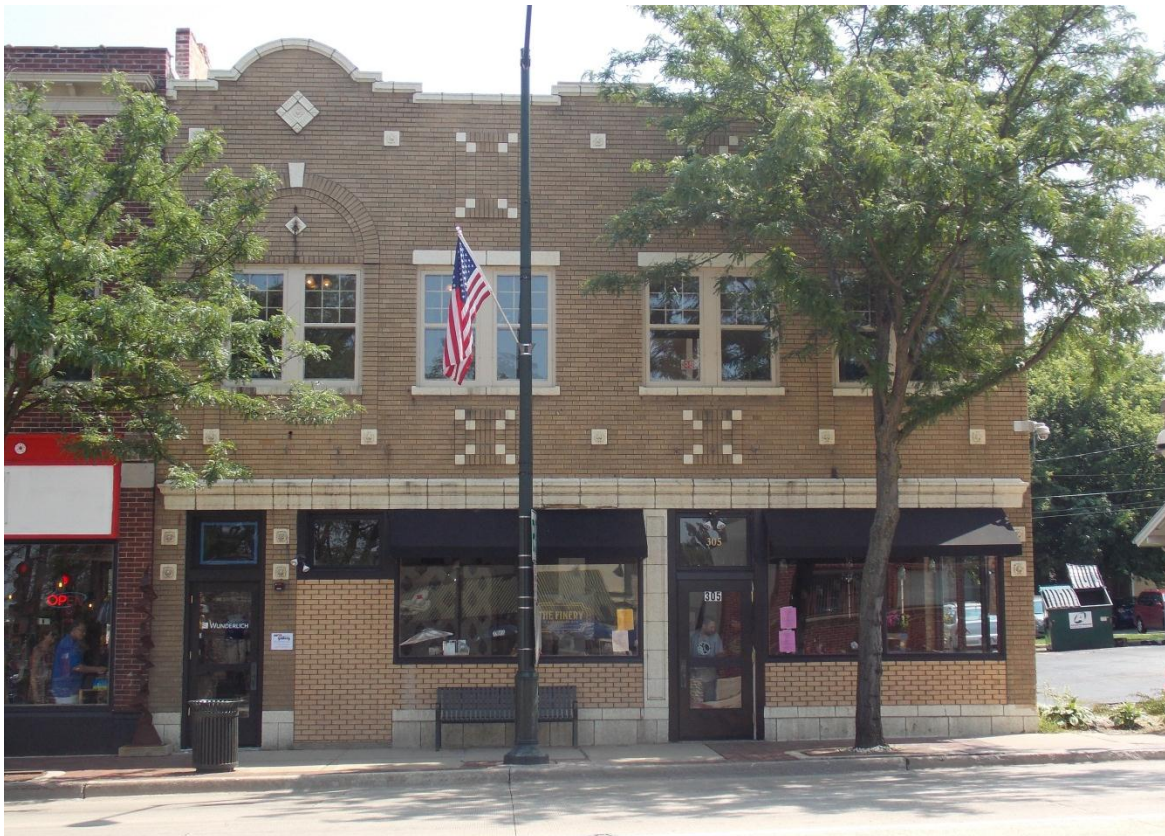
305 W Main St. - AFTER
