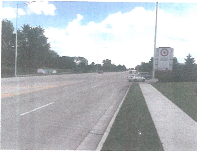
Looking south at access point off Kautz Road
