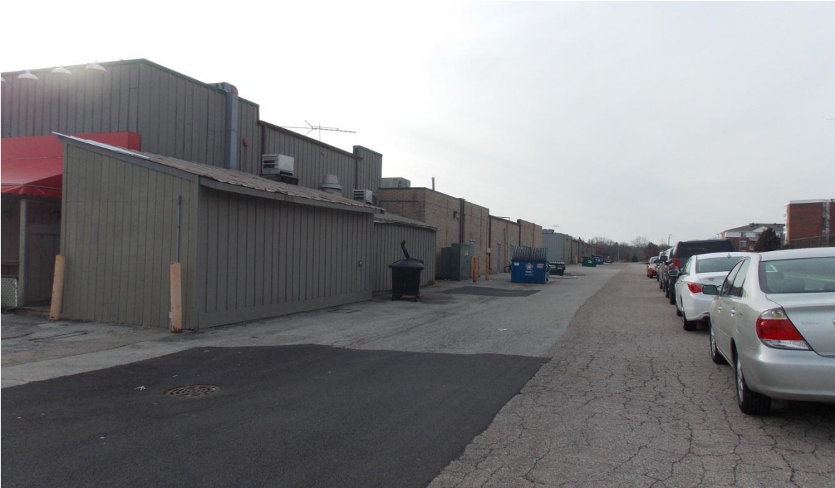
1. Drive-through lane location – rear of building (north side)
