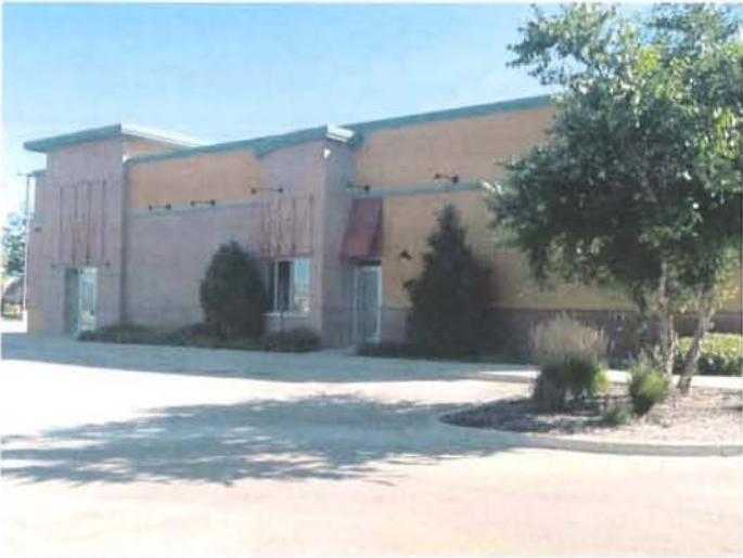
EXISTING SIDE ENTRANCE
