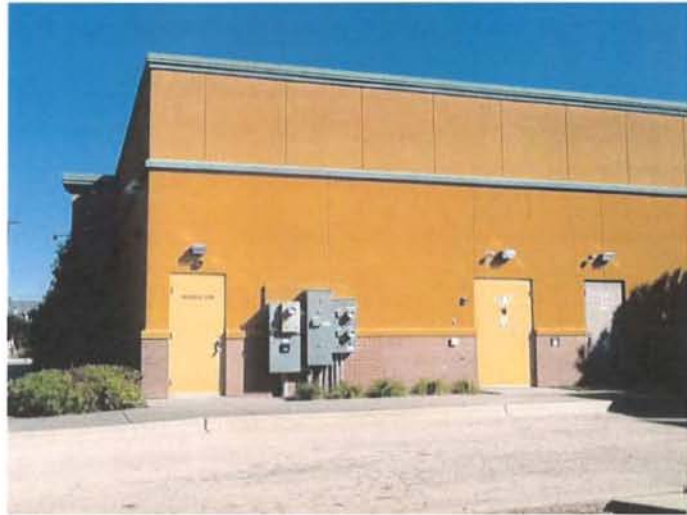
EXISTING REAR EXIT
