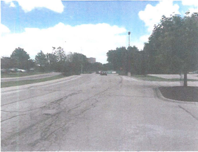
Looking east at access point off Kautz Road
